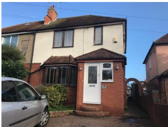
Photo 1: Southern elevation of the house
