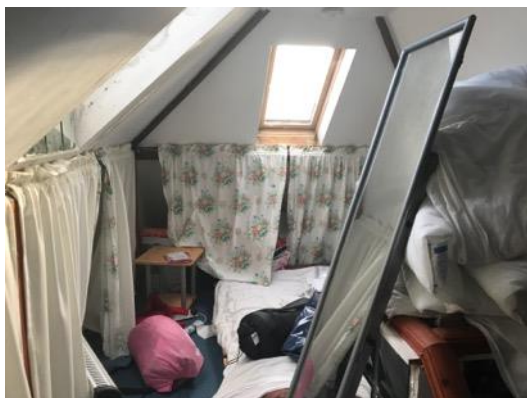
Photo 3: Internal loft space convert into living space
