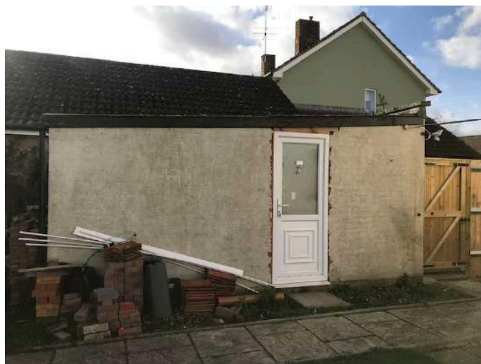
Plate 9: North Face of Garage
