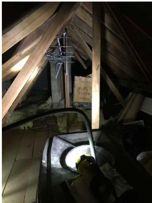
Plate 10: Internal Roof Void facing North
