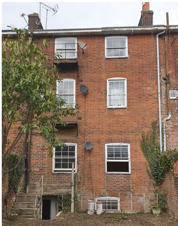
Figure 2:: 245 Oxford Rd-rear-Existing photograph
