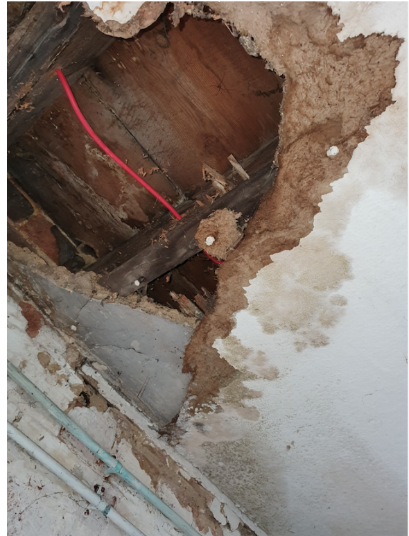
Figure 3: Ceiling of lower ground floor
