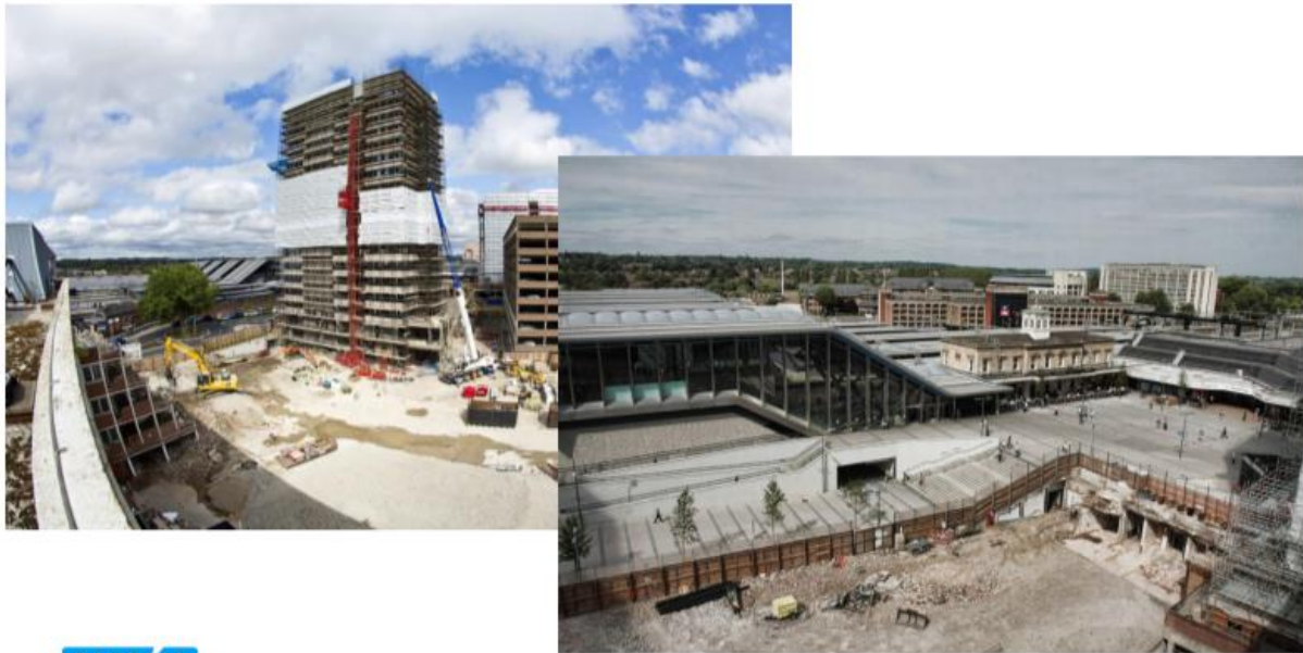
Figure 2: Historic photographs showing frame of Thames Tower and demolition site north of NCP car park.
