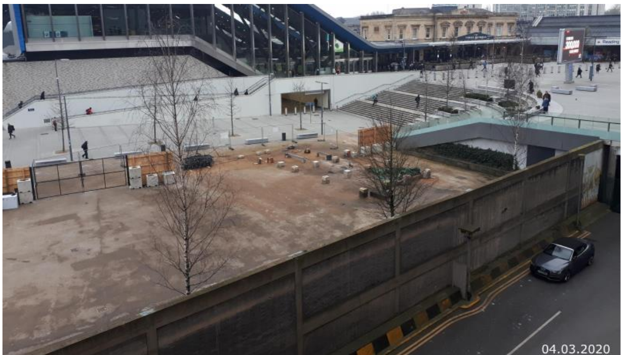
Figure 5: 2020 Phase 1 Enabling works site including existing retaining wall to NCP car park road
