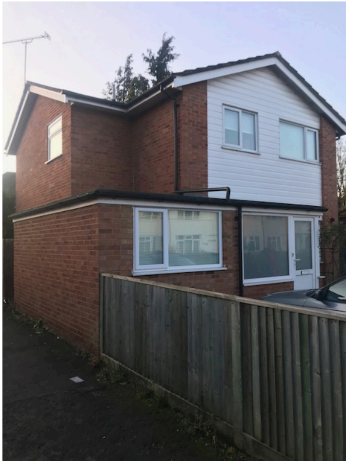
Photograph showing the front and south elevation of the house.
