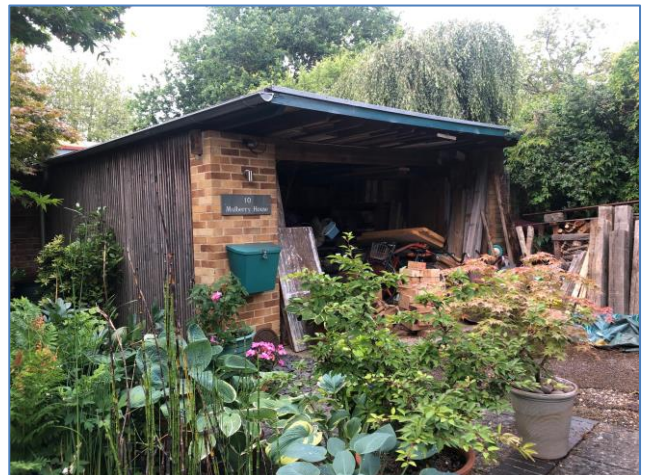
2. Existing Garage - 10 Ridge Hall Close
