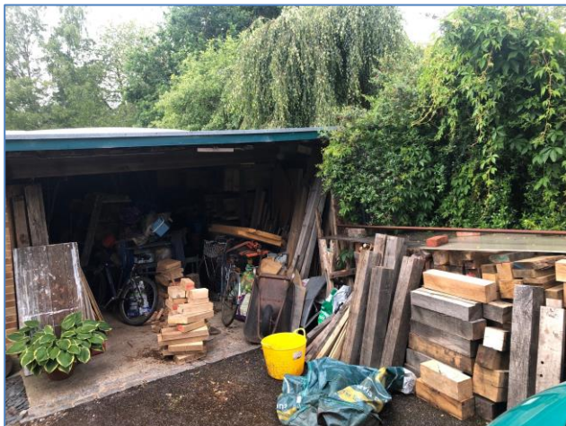
1. Existing garage - 10 Ridge Hall Close
