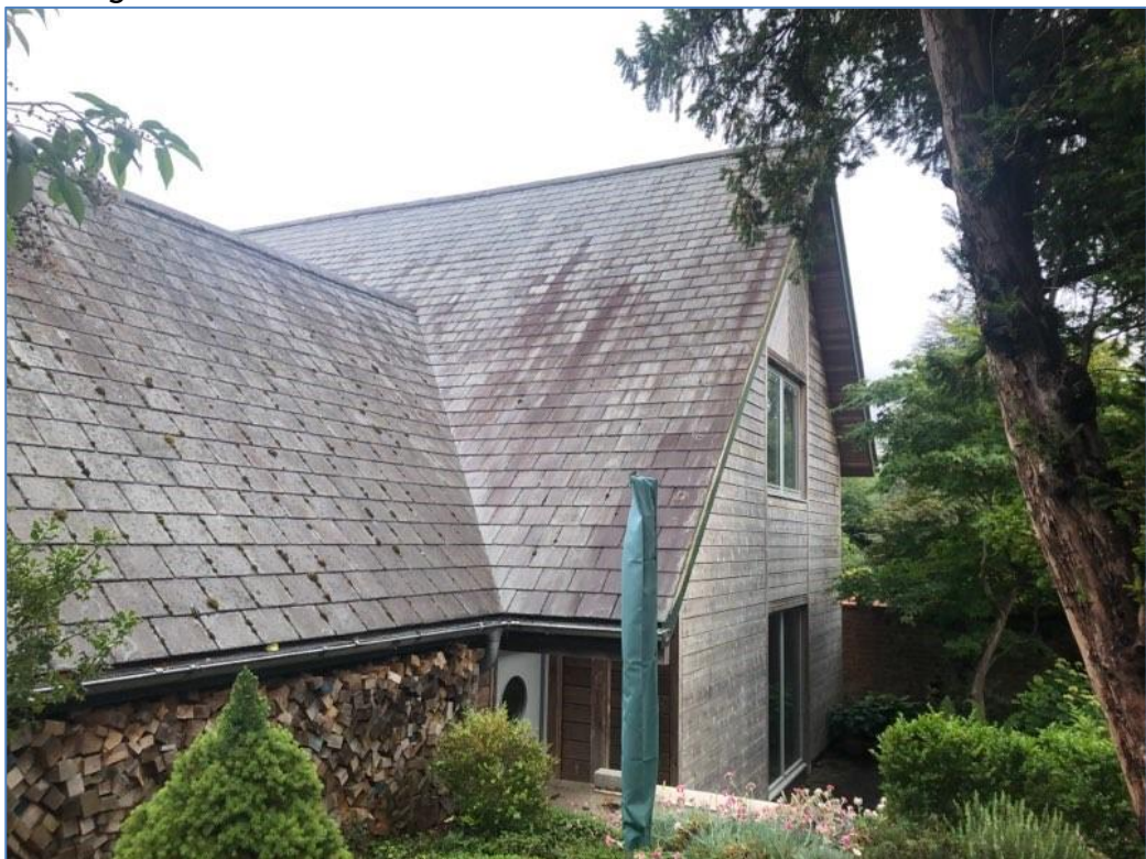
3. Roof of the existing dwelling house 10 Ridge Hall Close.
