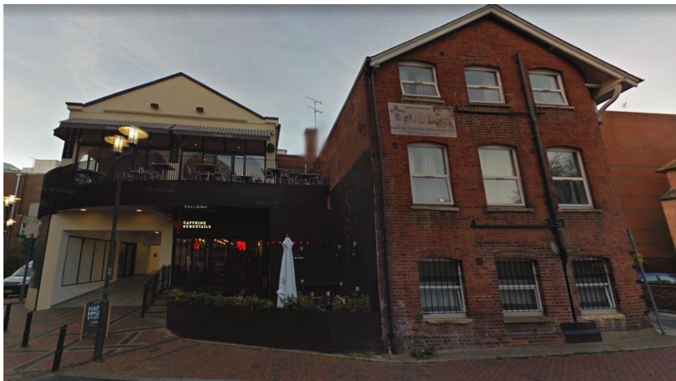
Figure 1.3: Existing Outdoor Sitting Area
