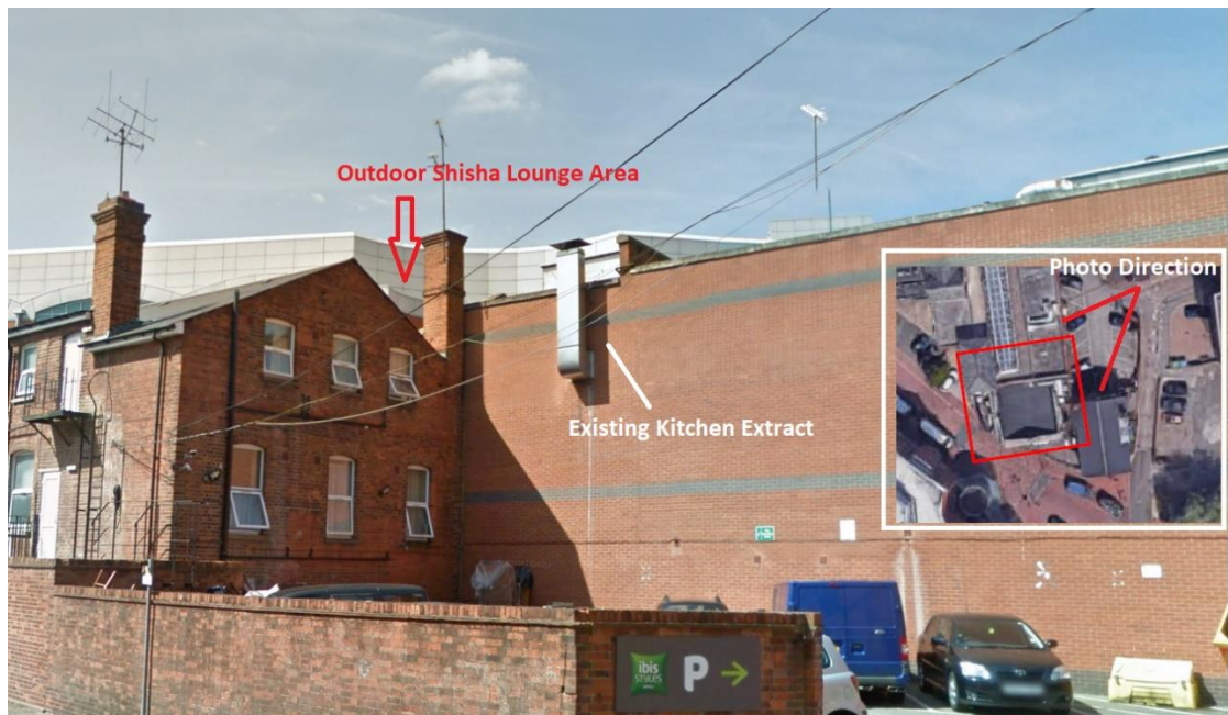
Figure 1.2: Existing Kitchen Extract
