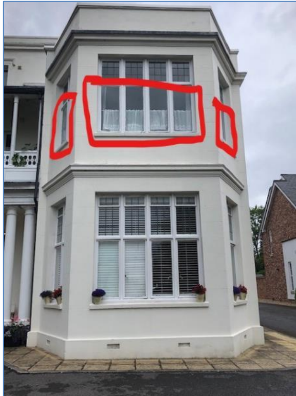
Fig 1. First floor windows highlighted in red to be replaced.
