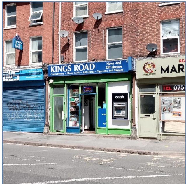
2. Existing Elevations. Photo taken on 12/05/2020.
