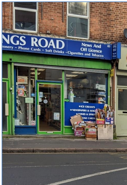
1. Pre-Existing Elevations. Photo taken on 05/12/2019.
