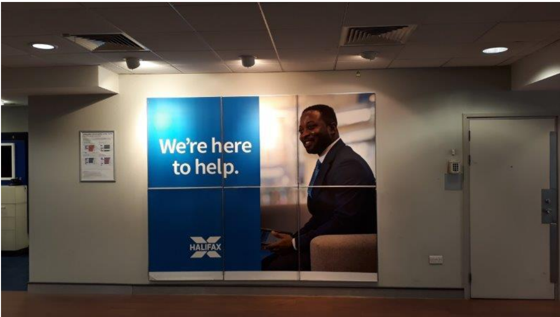
General internal finishes and fit out to be replaced.
