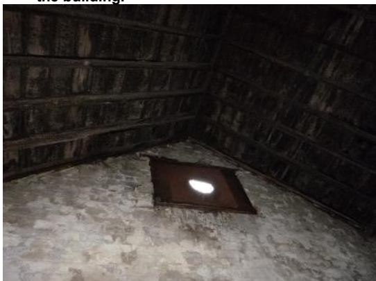
11. An opening to the exterior in the southern gable wall of the slate covered roof.
