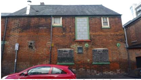
1. The building viewed from St John's Street to the east looking west.
