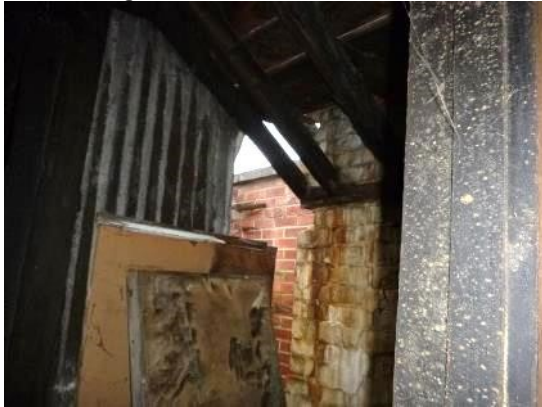
15. An opening to the exterior at the building's south western corner.
