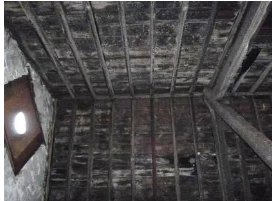
10. The timber sarking lining the slate roof on the building's eastern side.
