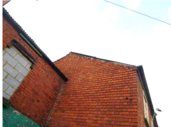
4. The southern gable end of the lower level, corrugated sheet roofed section of the building.
