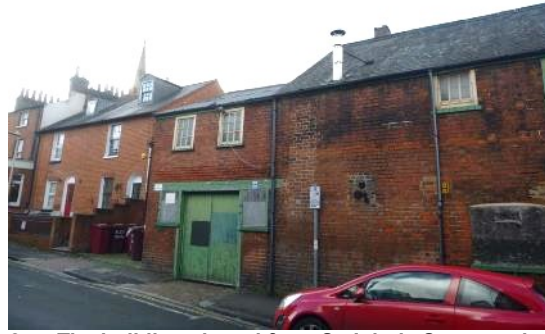
2. The building viewed from St John's Street to the east looking south west showing lower level corrugated sheet covered roof.
