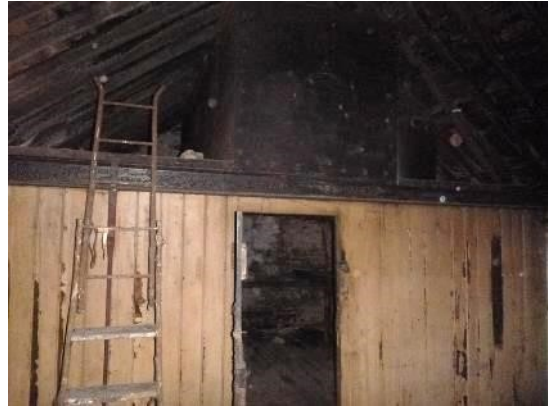
14. The raised water tank and room beneath on the western side of the building.
