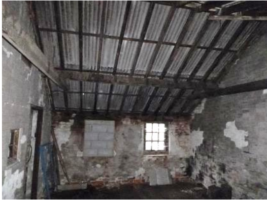
7. The corrugated sheet roof on the eastern side of the building.
