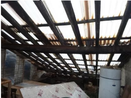
9. Corrugated sheet roof on the western side of the building.
