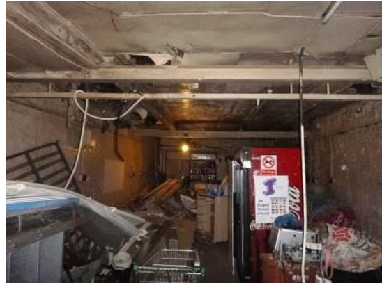
16. The storage space on the building's ground floor.
