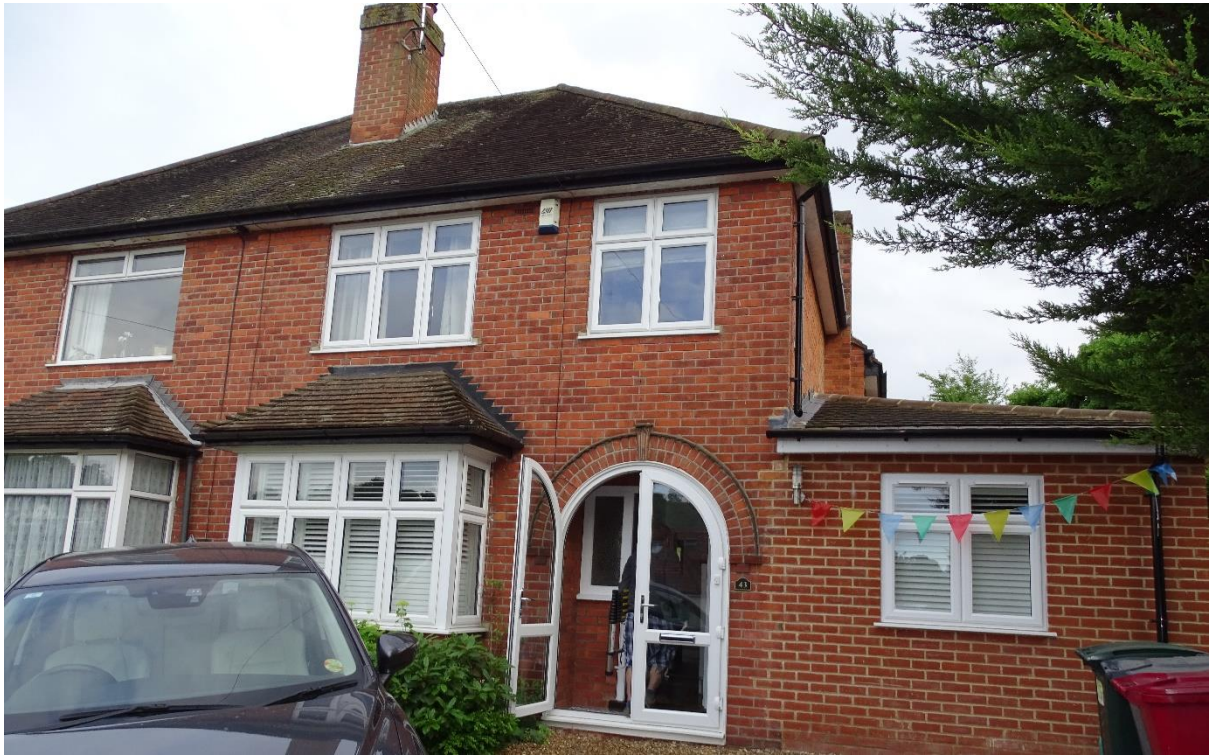
Image 1 – Front North facing elevation of the property
