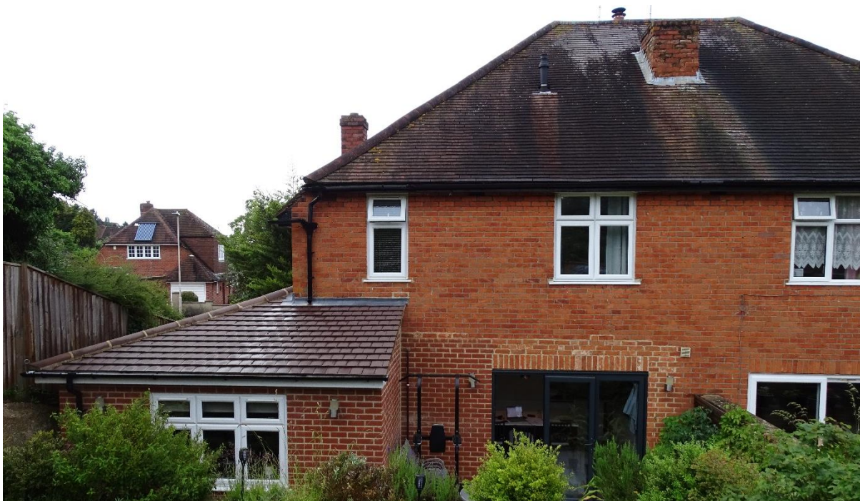
Image 4 – Rear South facing elevation of the property
