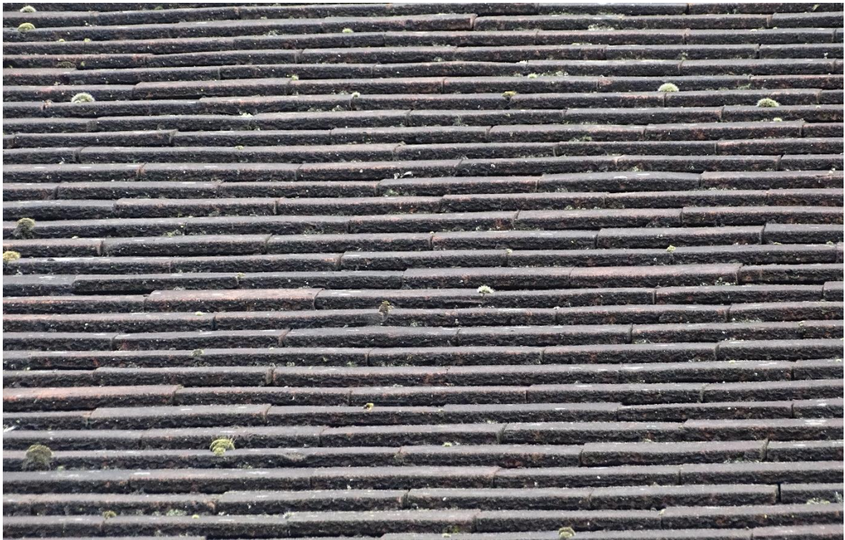
Image 5 – Close view of roof coverings across the West facing elevation which have demonstrated a fair condition throughout
