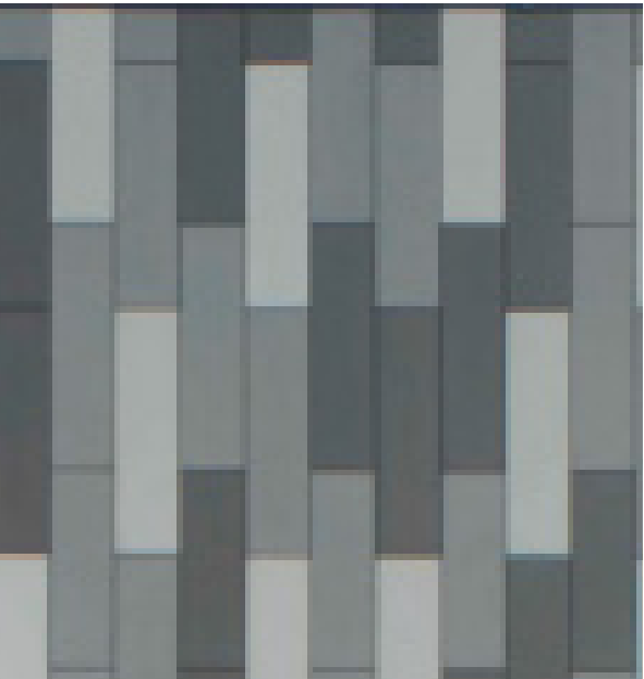
Rock panel cladding
