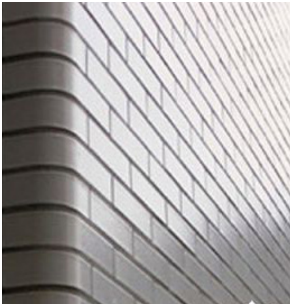
White glazed brick to balcony recesses
