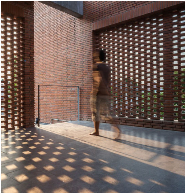
Perforated brick screening to the car park area
