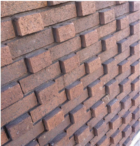
Patternated brick work
