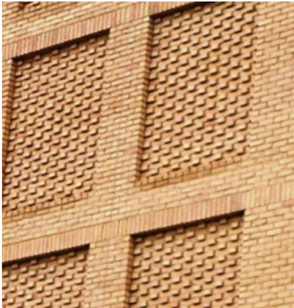
Recessed brick panels with patternated brickwork
