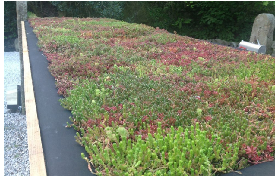
Green Sedum roof
