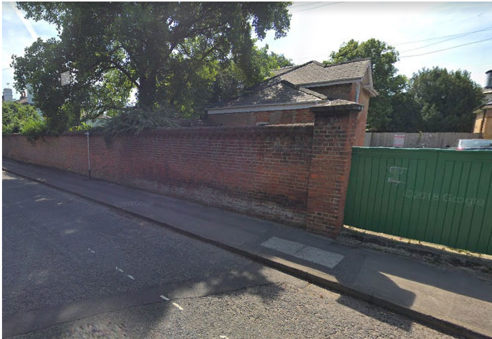
Above: Existing wall along the site boundary on Upper Redlands Road
