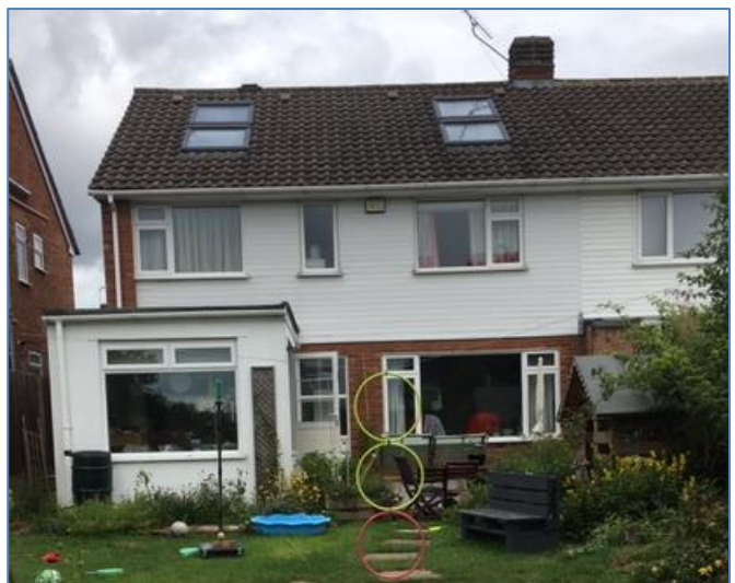
2. Rear elevation of 23 The Ridgeway (image supplied by applicant).
