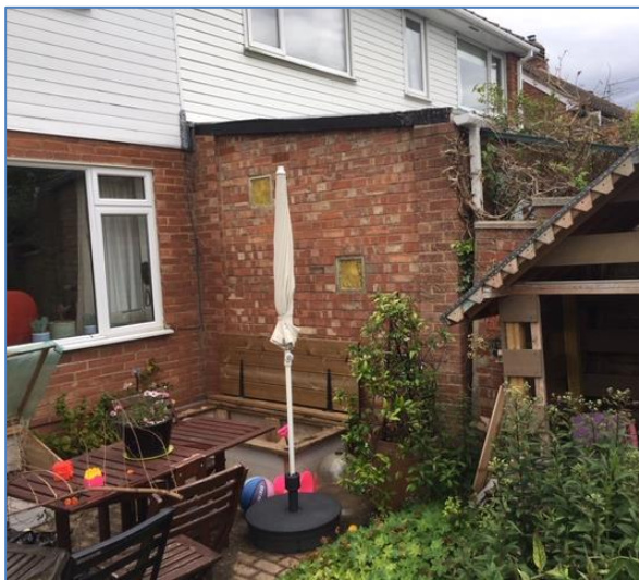
1. Rear extension to 21 The Ridgeway (image supplied by applicant).
