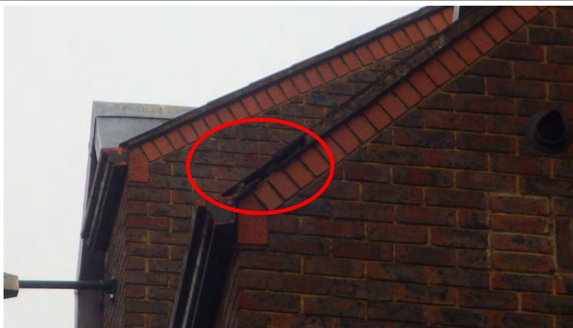
Photograph 9: A potential roosting feature (TN5) on the south-western elevation of building B2.
