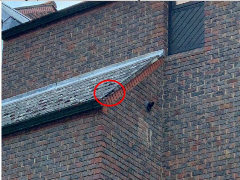
Photograph 2: PRF 2 on the lower level roof
