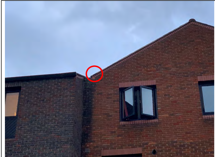
Photograph 1: PRF 1 on the western gable
