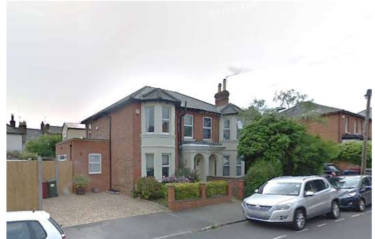
View of No 7 Eastern Avenue – property located opposite of the application site
