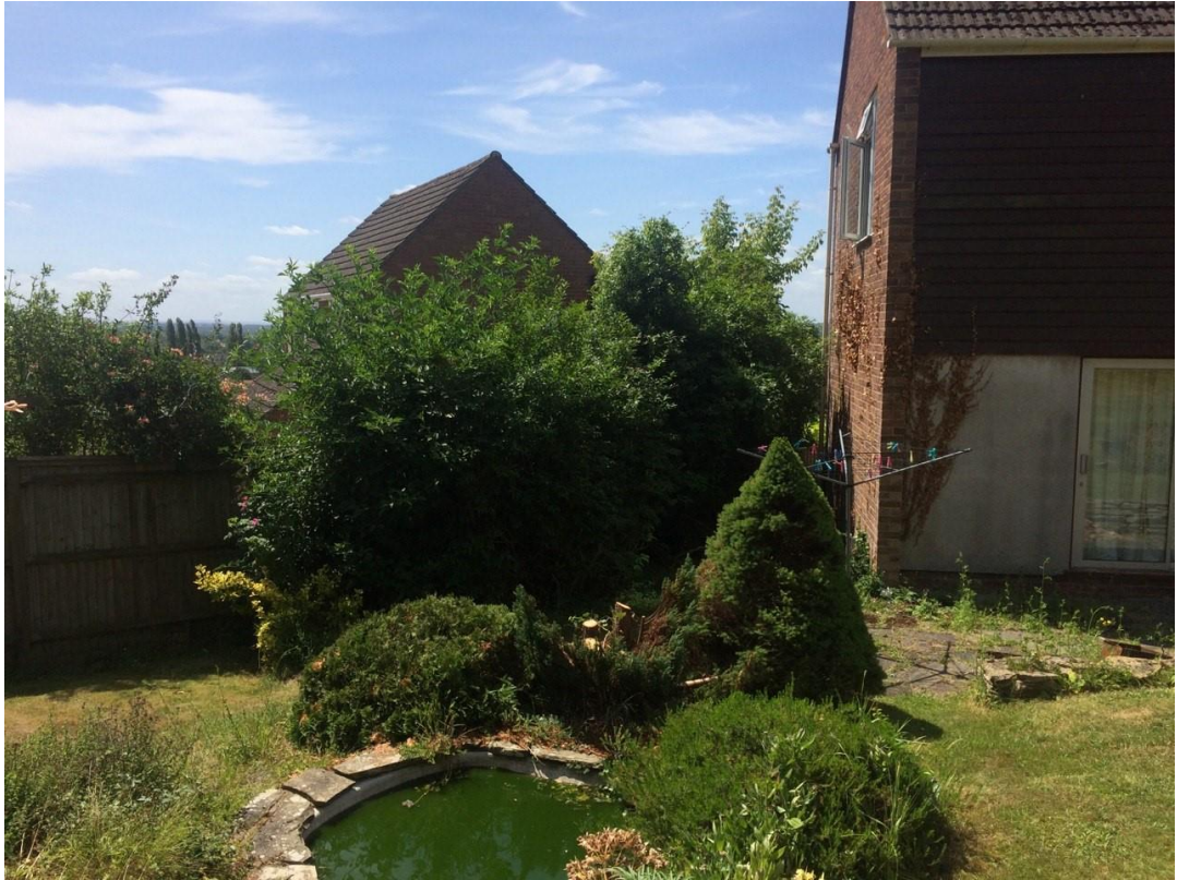
2. Existing Rear Elevation - 36 Fontwell Drive. 34 Fontwell Drive also pictured.
