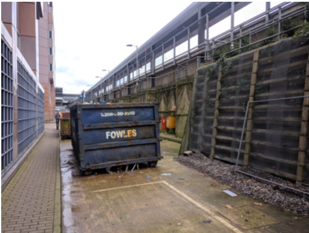
View at basement level
