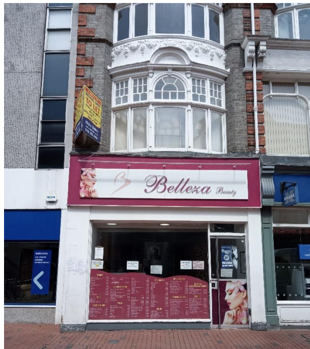
1. Existing Elevations. Photo taken on 12/05/2020.
