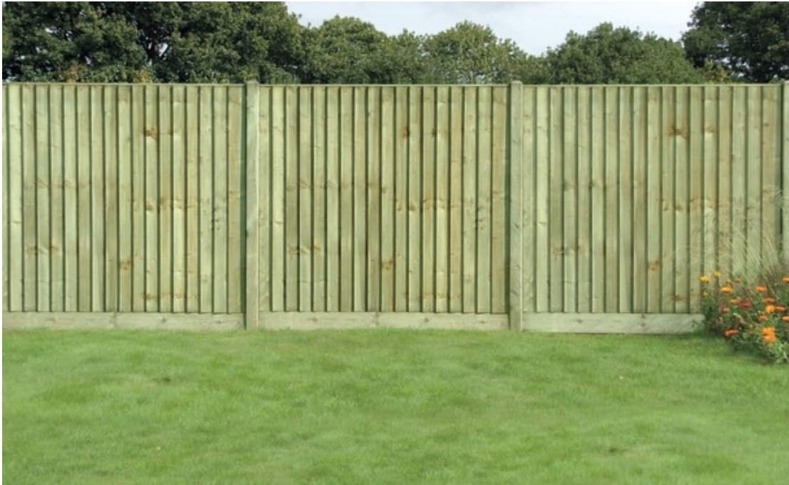
Close board fencing
