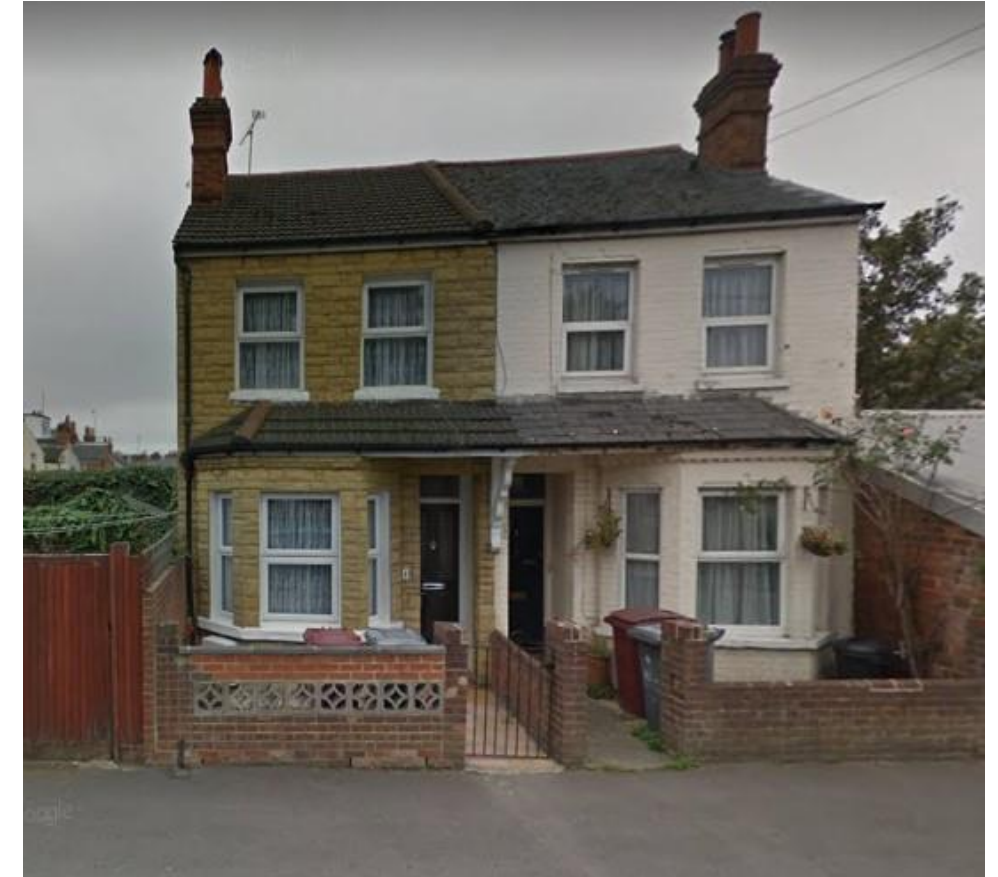
Figure 4 Existing semi-detached dwellings on Gordon Place
