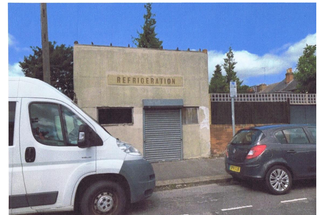
Figure 3 Existing building on the site to be demolished
