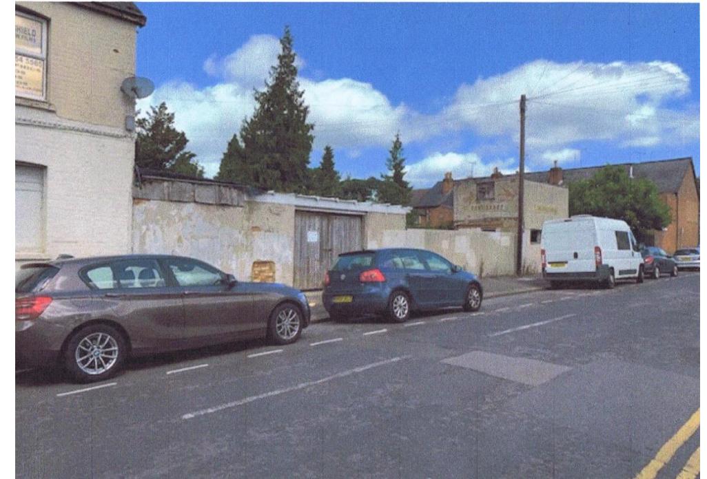
Figure 2 View of the site from Gordon Place
