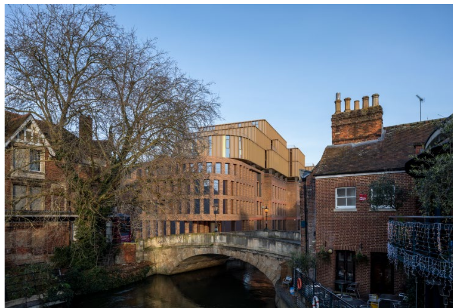
View from yield hall place bridge, looking east
