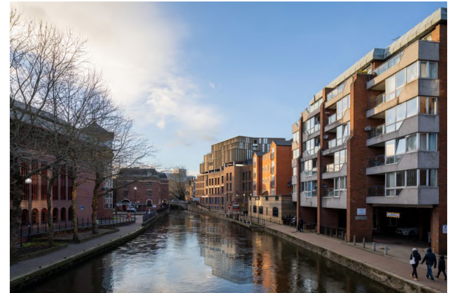
View from footbridge across river kennet south of crane wharf looking west
