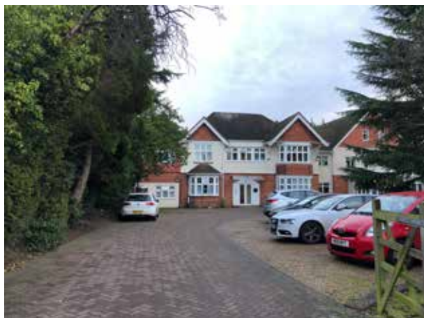
View of entrance to the site showing building and extensions
