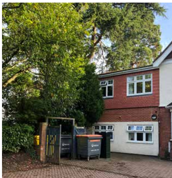
Existing bin store in close proximity to bedroom windows
