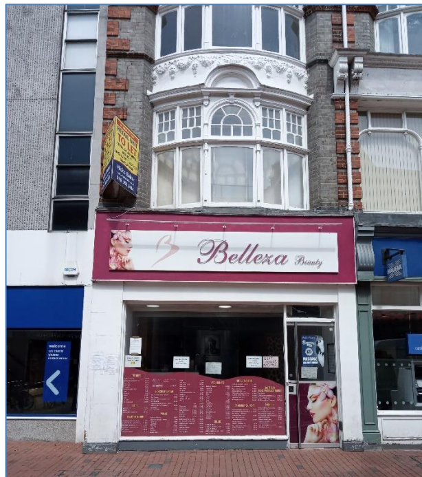
1. Existing Elevations. Photo taken on 12/05/2020.
