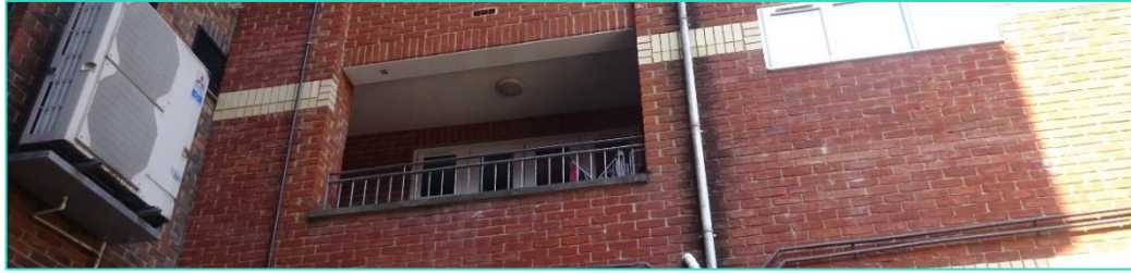
Extract 03: Site Photograph LK R1/111 (Served by W1/111, W2/111 and W3/111)
