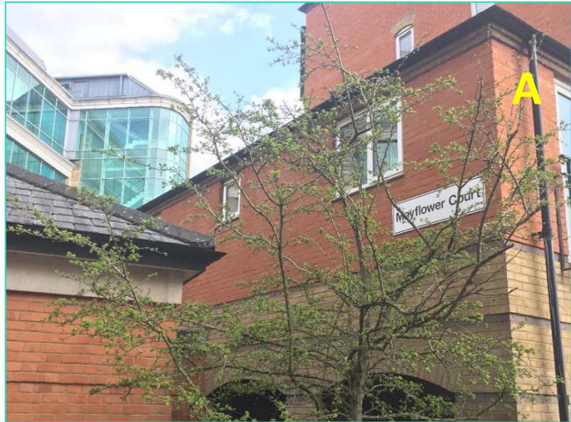
Extract 07: Site photograph; side elevation of Mayflower Court
