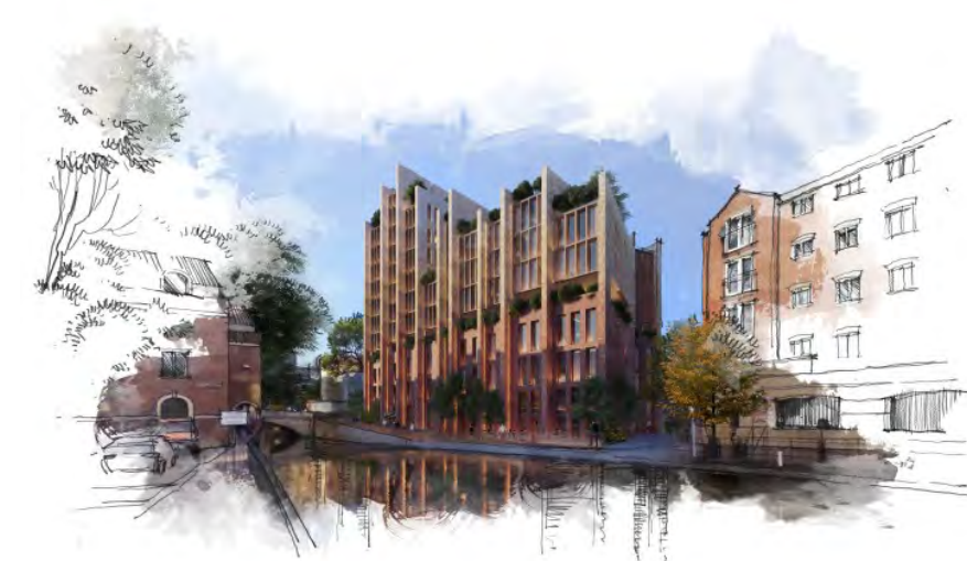
A fourteen storey tall building on the west corner that gradually steps down towards the east end with a graded brick that starts from the existing red and lightens towards the top
