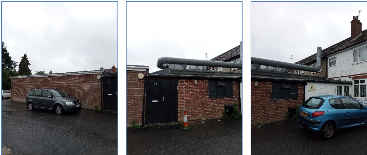
1. Side elevations to the rear of 6 Park Lane. Photos taken on 19/08/2020.
