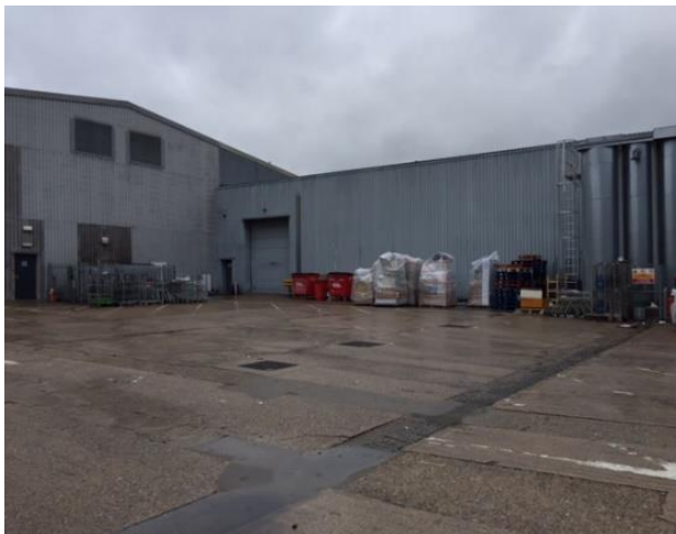
North-west facing view from behind commercial units in the south of the application site
