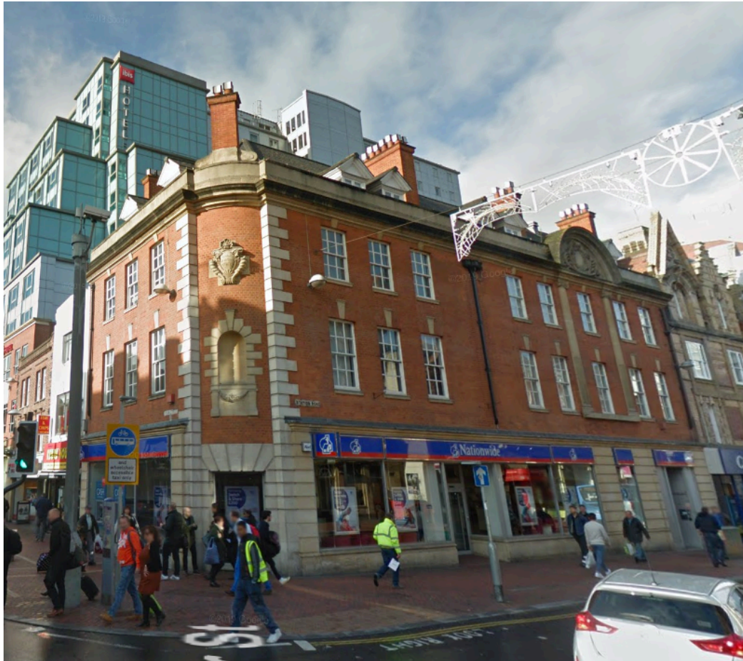
External image of the site (Google Street View)
