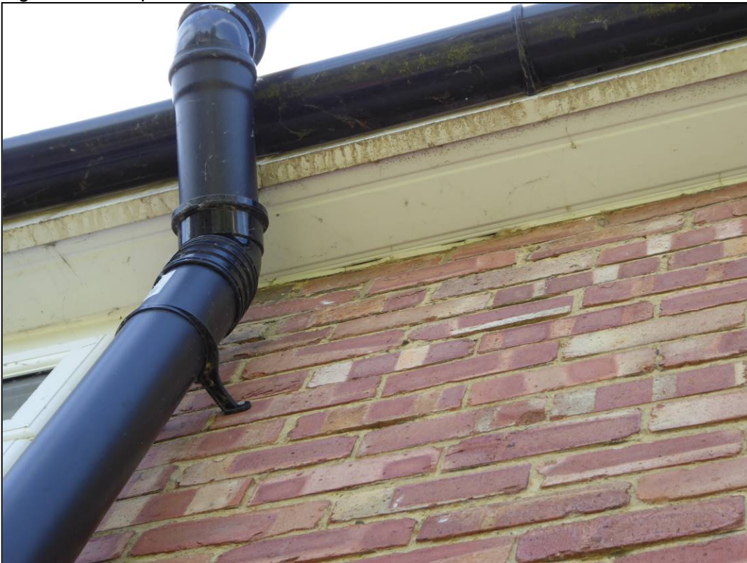
Figure 6. Example of soffits. 12 Mill Green, Caversham. 18.05.20
