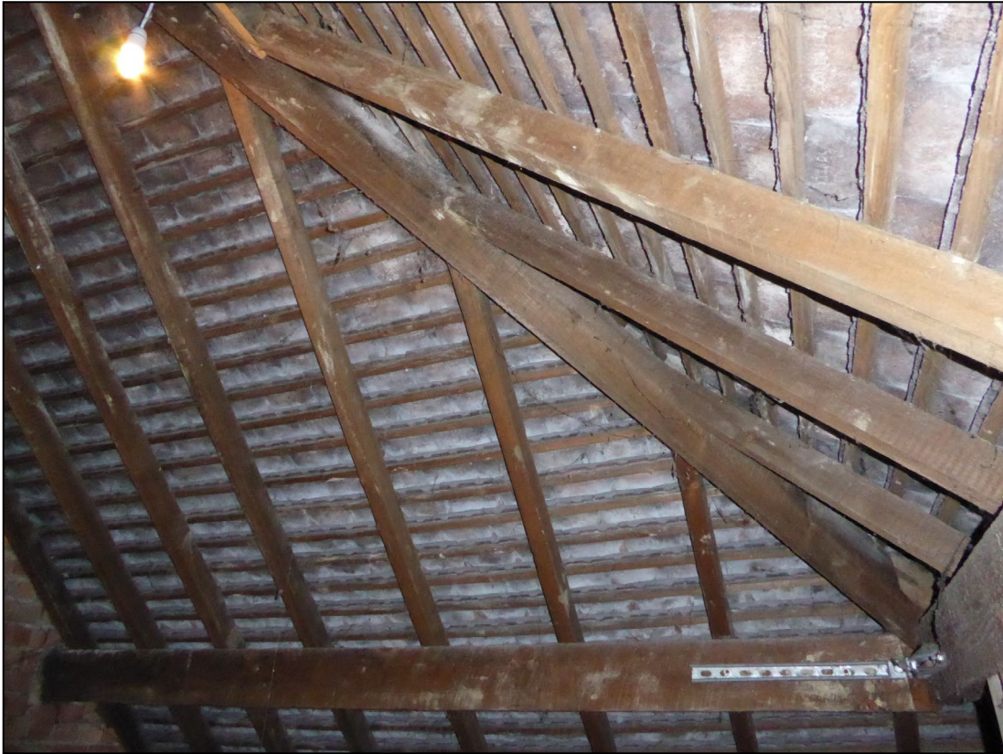
Figure 10. Unlined roof tiles. 12 Mill Green Caversham. 18.05.20
