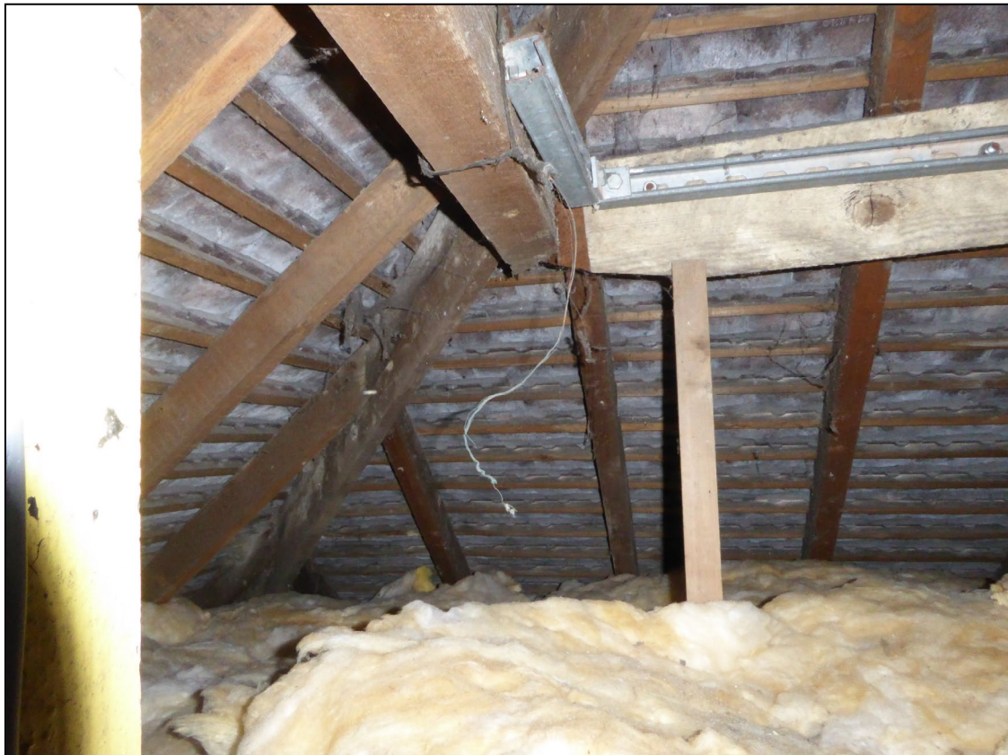
Figure 9. Loft space. 12 Mill Green Caversham. 18.05.20
