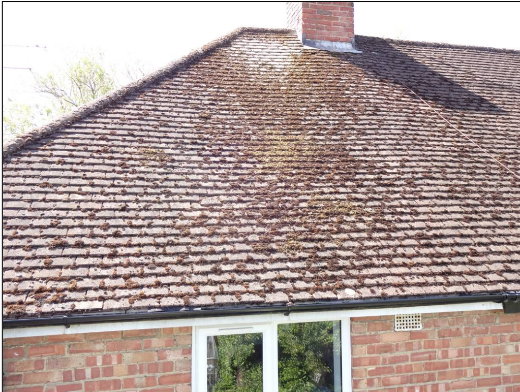
Figure 4. Example of roof tiles. 12 Mill Green, Caversham. 18.05.20
