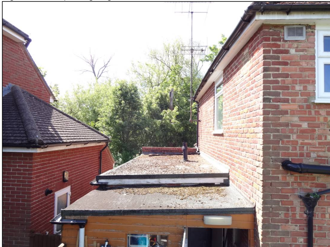
Figure 8. Example of garage roof. 12 Mill Green, Caversham. 18.05.20
