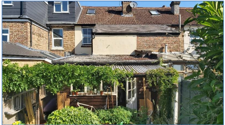
2. Existing rear elevation of 24 Junction Road.
