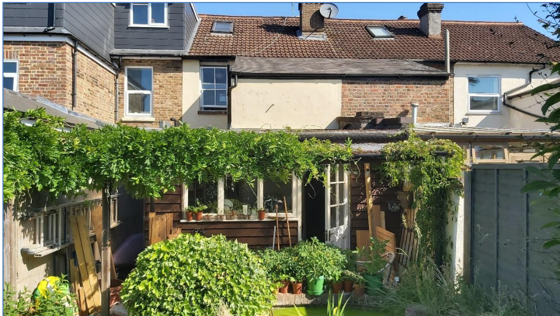
1. Rear of 24 Junction Road. Photo provided by the agent on 28/07/2020.
