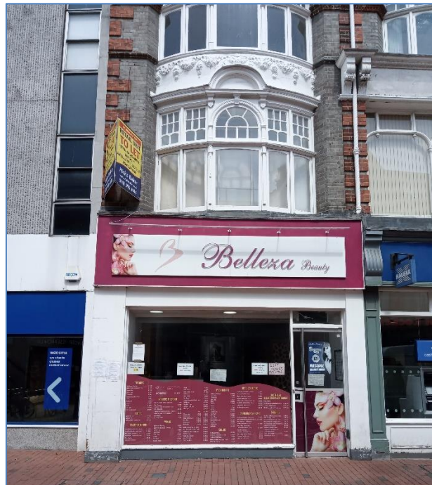
1. Existing Elevations. Photo taken on 12/05/2020.
