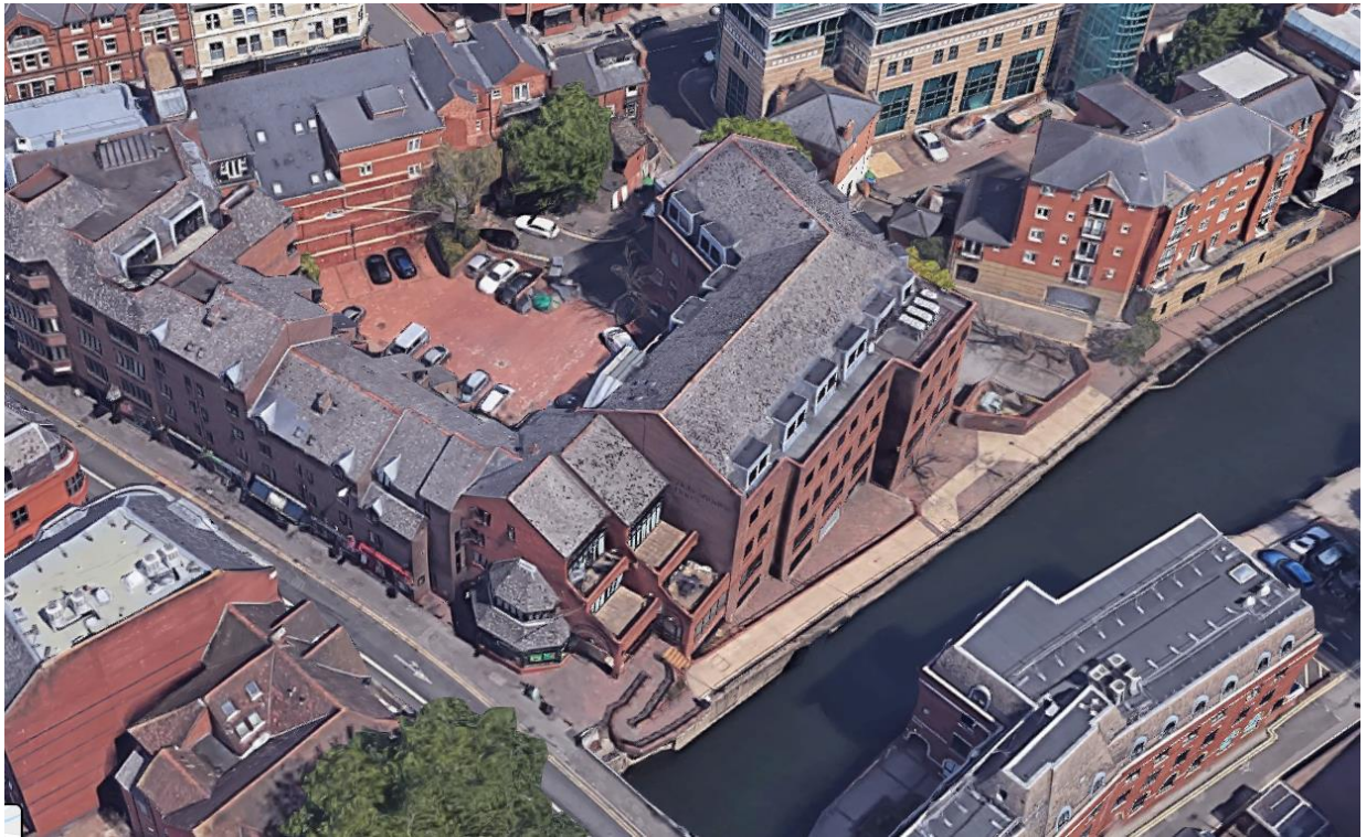
Figure 5: Photograph of Dukesbridge House from the South-west
