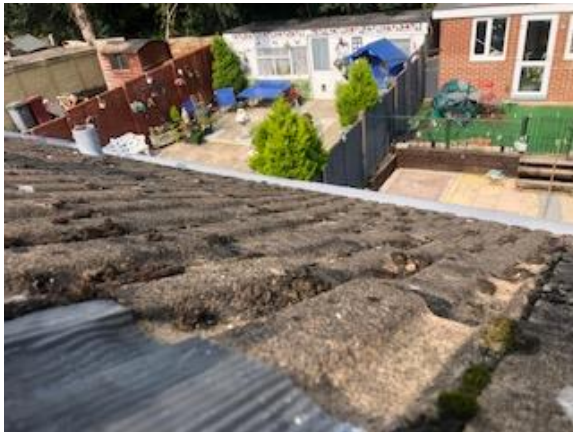
View out of Velux window, intact plastic flashing around window and tight and intact cement tiles
