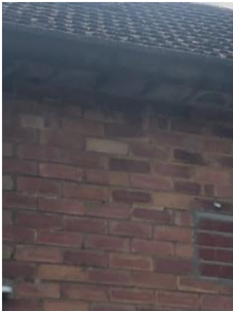
Intact cement 'soffits' at rear
