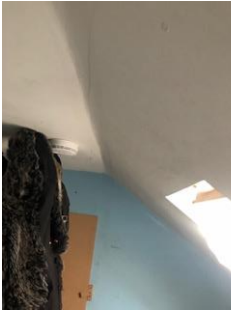
Roof space of converted loft space
