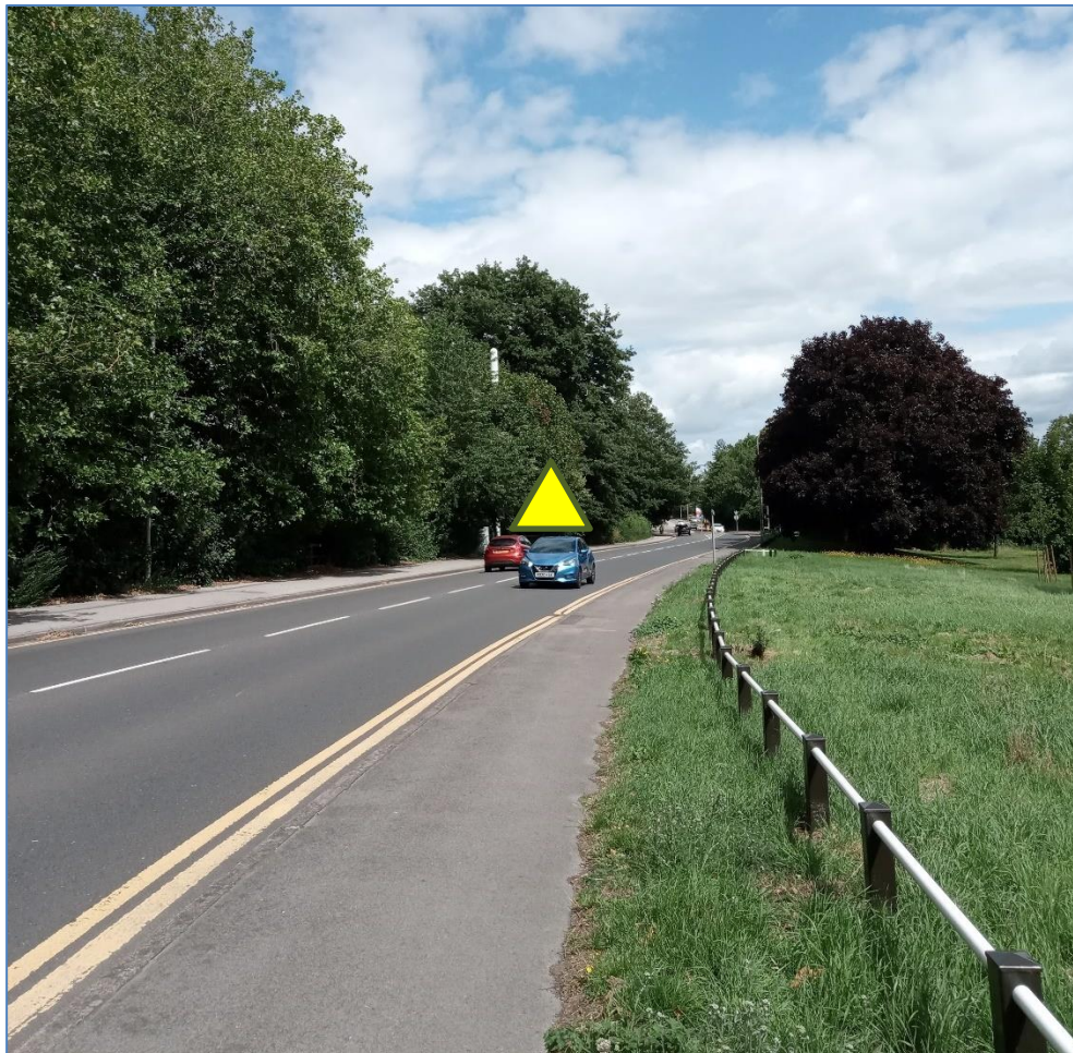
Fig 3. Viewing Angle 1, heading eastbound along Bath Road. Photo taken on 06/07/2020.
