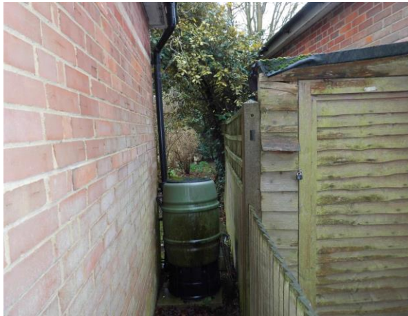
Rear of detached garage.
