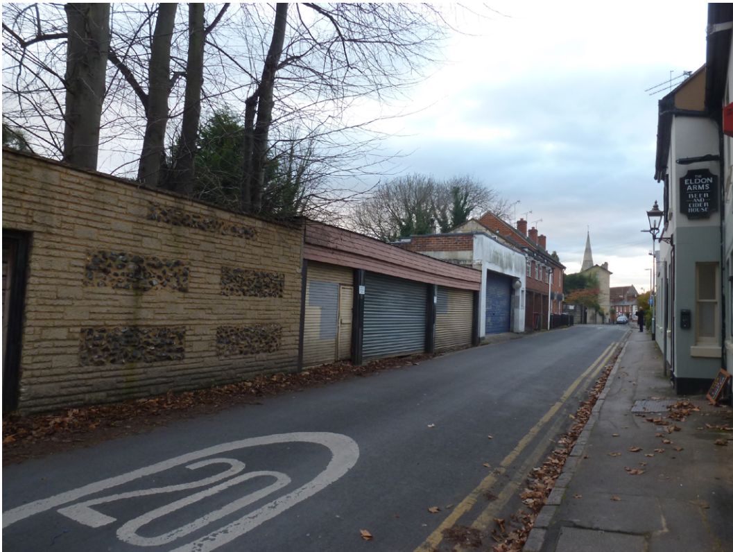
Fig.1: Photograph looking west along Eldon Terrace of previous garage buildings on application site (now demolished)
