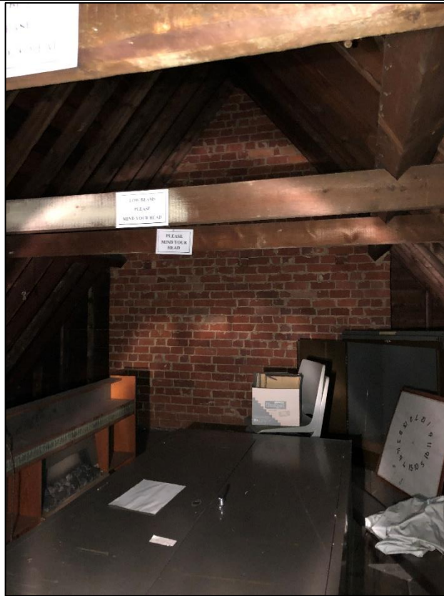
Figure 9: Void A, boarded and used for storage
