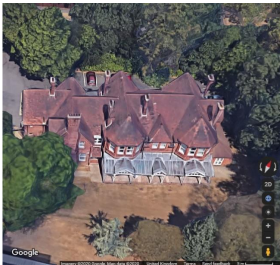
1. Existing Elevations. Image retrieved from Google Maps on 29/05/2020.
