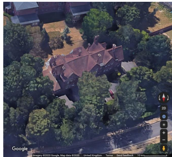
2. Existing Elevations. Image retrieved from Google Maps on 29/05/2020.
