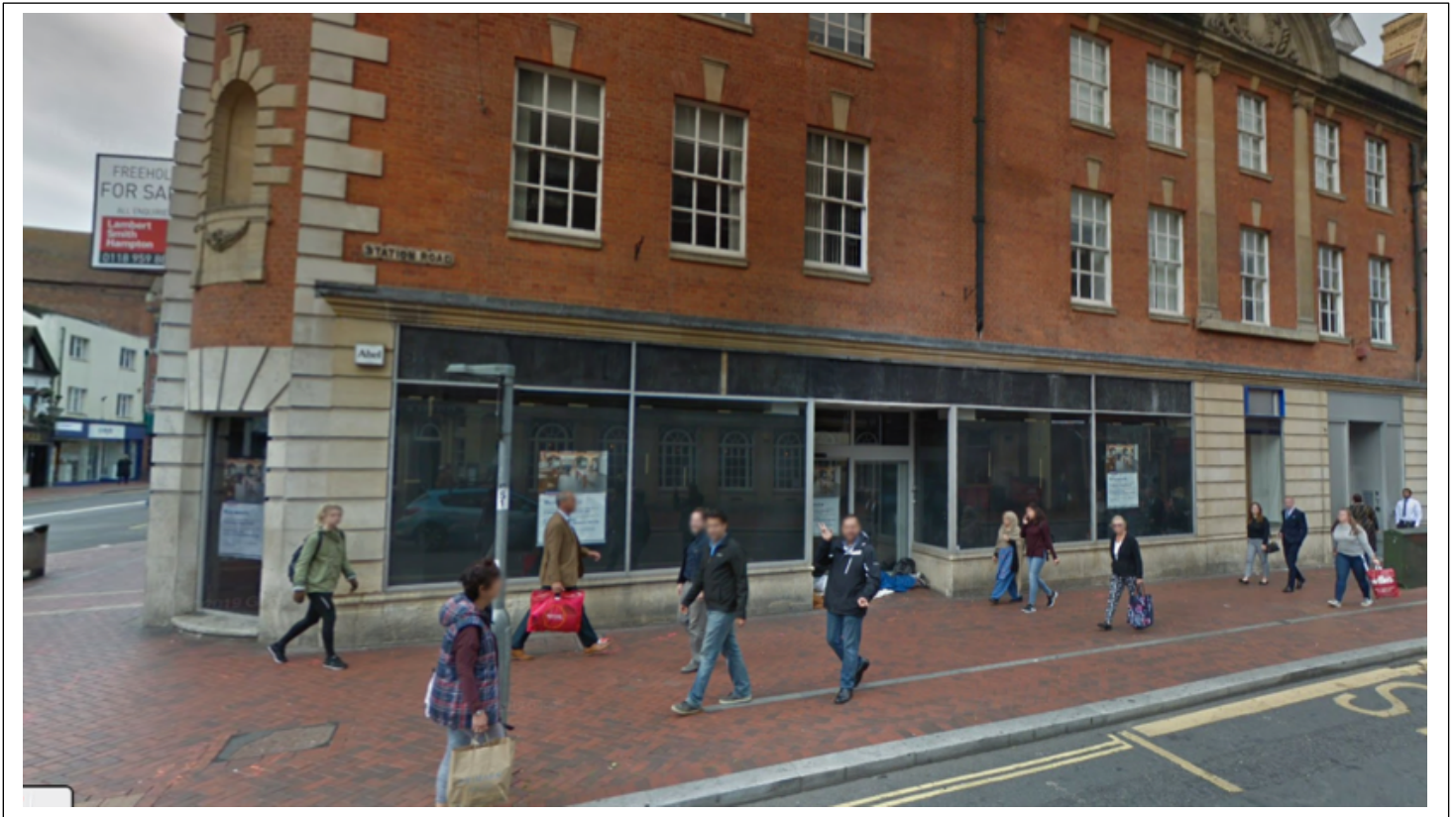
‘As Existing’ Station Road:
