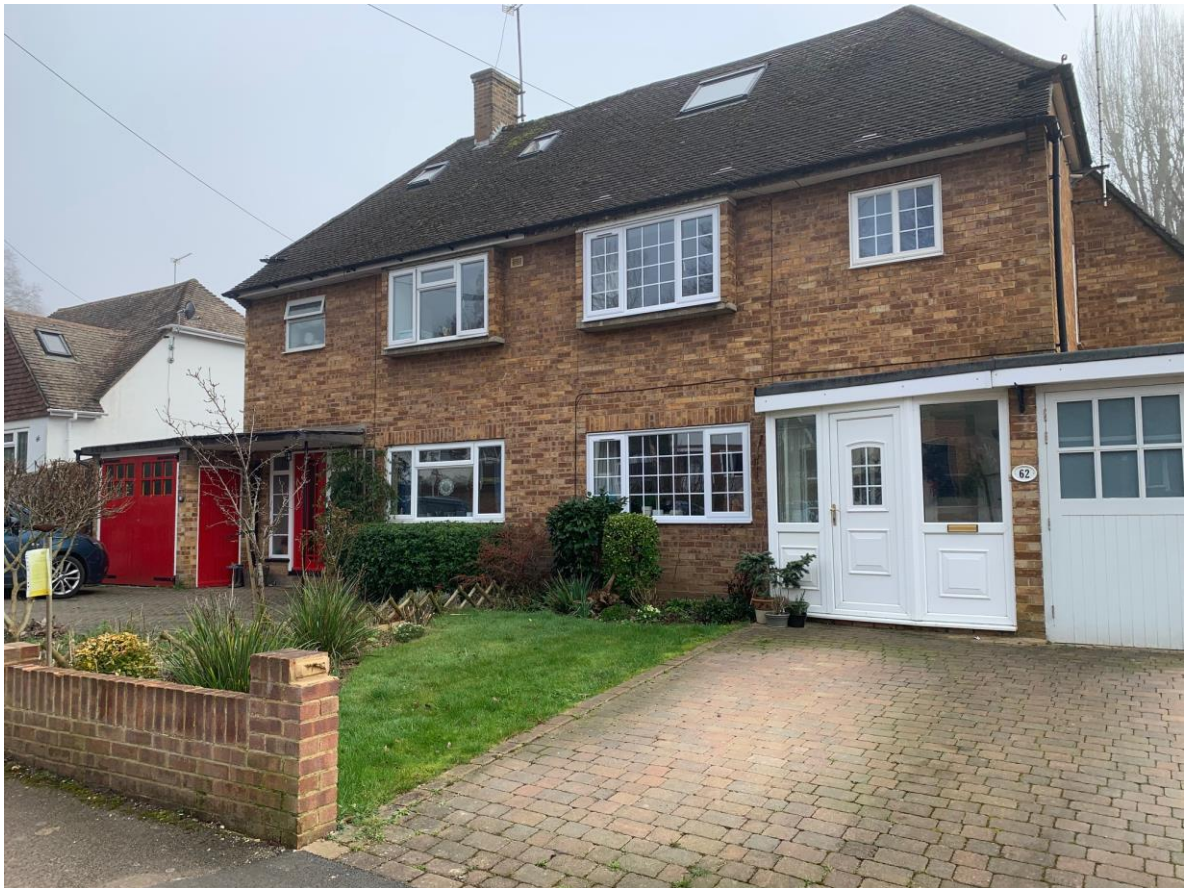
View of the front/north elevation in the context of being a semi-detached dwelling.
