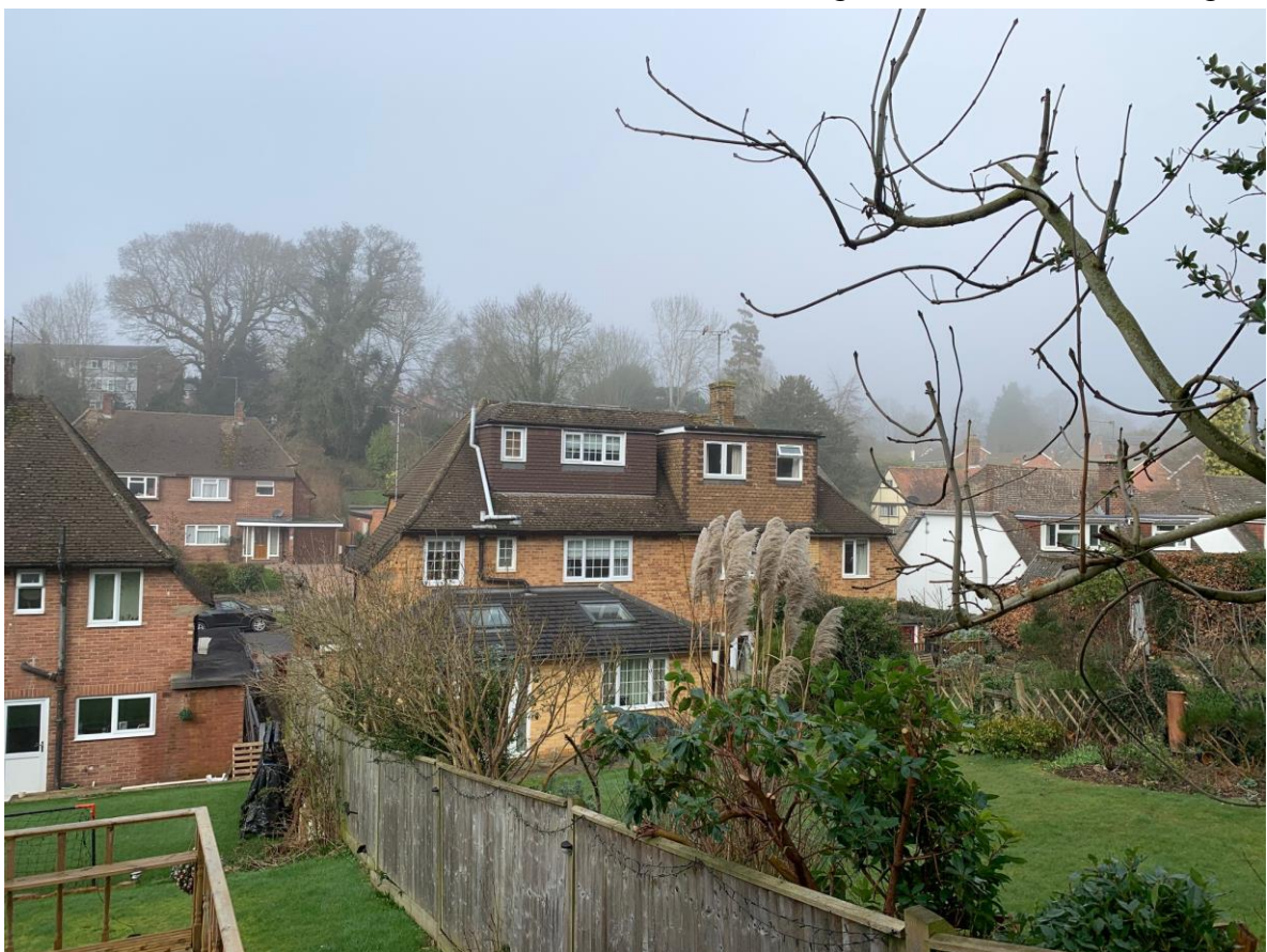
A view of the rear/south elevation as viewed from the end of 60 Rotherfield Way's garden.
