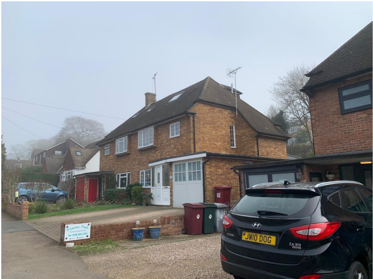
View of the side/west elevation as viewed from the street.
