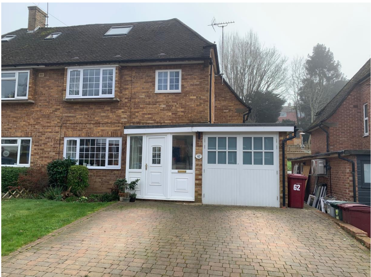
View of the front/north elevation; note the receding/angled porch and flat roof.
