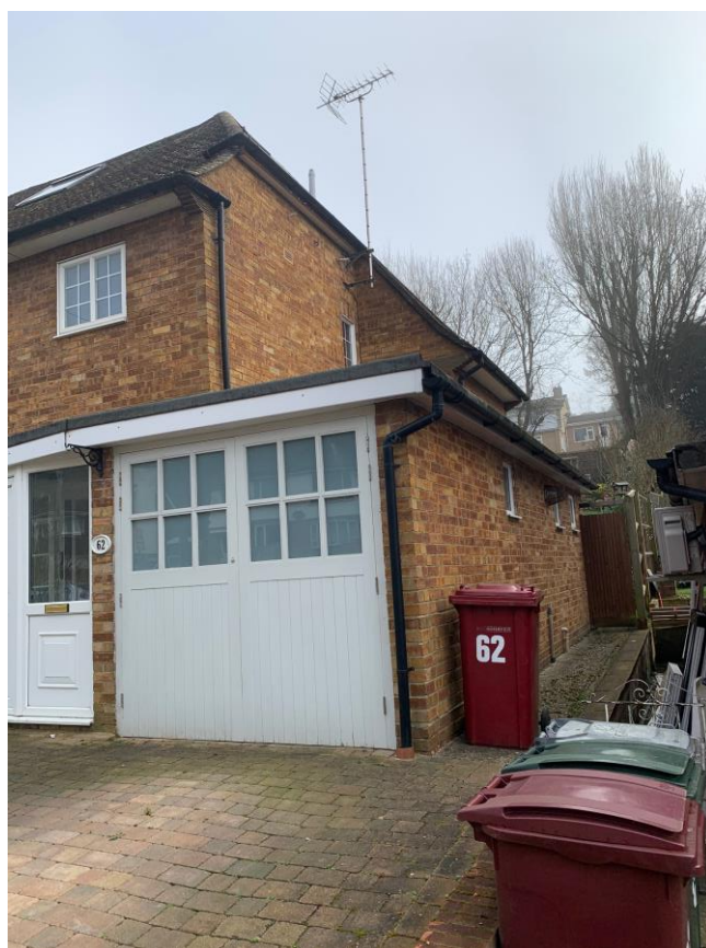
A view of the side/west elevation and the boundary treatment with 60 Rotherfield Way.
