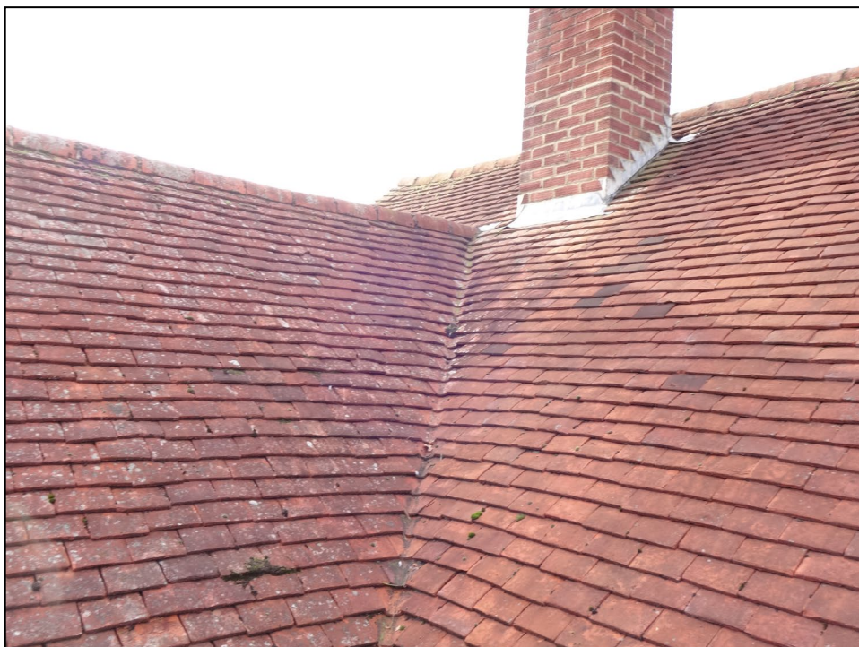
Figure 5. Sealed ridges, valleys and lead flashing. 132 Cockney Hill, Tilehurst. 24.11.20
