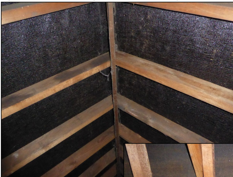
Figure 10. Bitumen lining to tiles. 132 Cockney Hill, Tilehurst. 24.11.20
