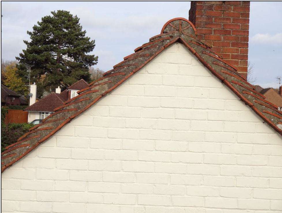
Figure 6. Sealed verges. 132 Cockney Hill, Tilehurst. 24.11.20
