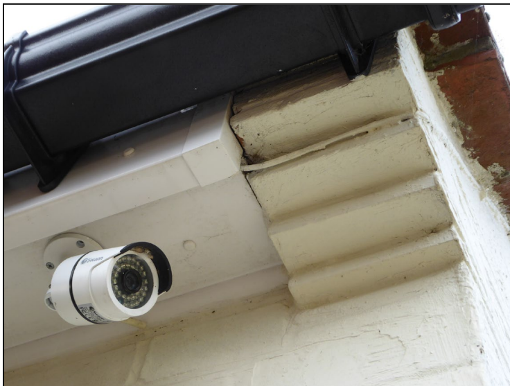
Figure 7. Sealed uPVC soffits and fascia's. 132 Cockney Hill, Tilehurst. 24.11.20
