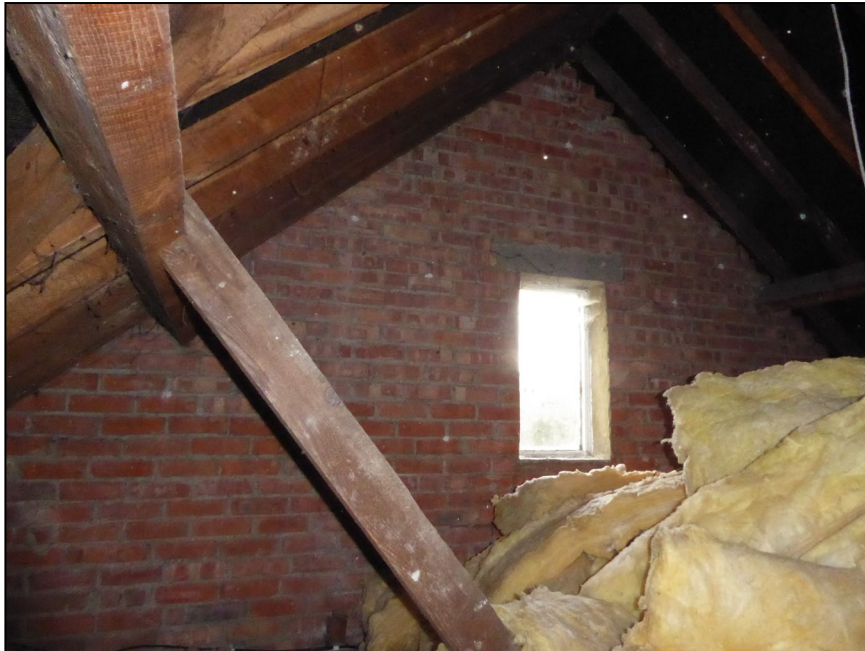
Figure 8. Windows at gable ends. 132 Cockney Hill, Tilehurst. 24.11.20
