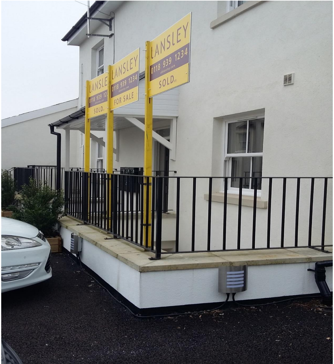
Existing front lightwells
