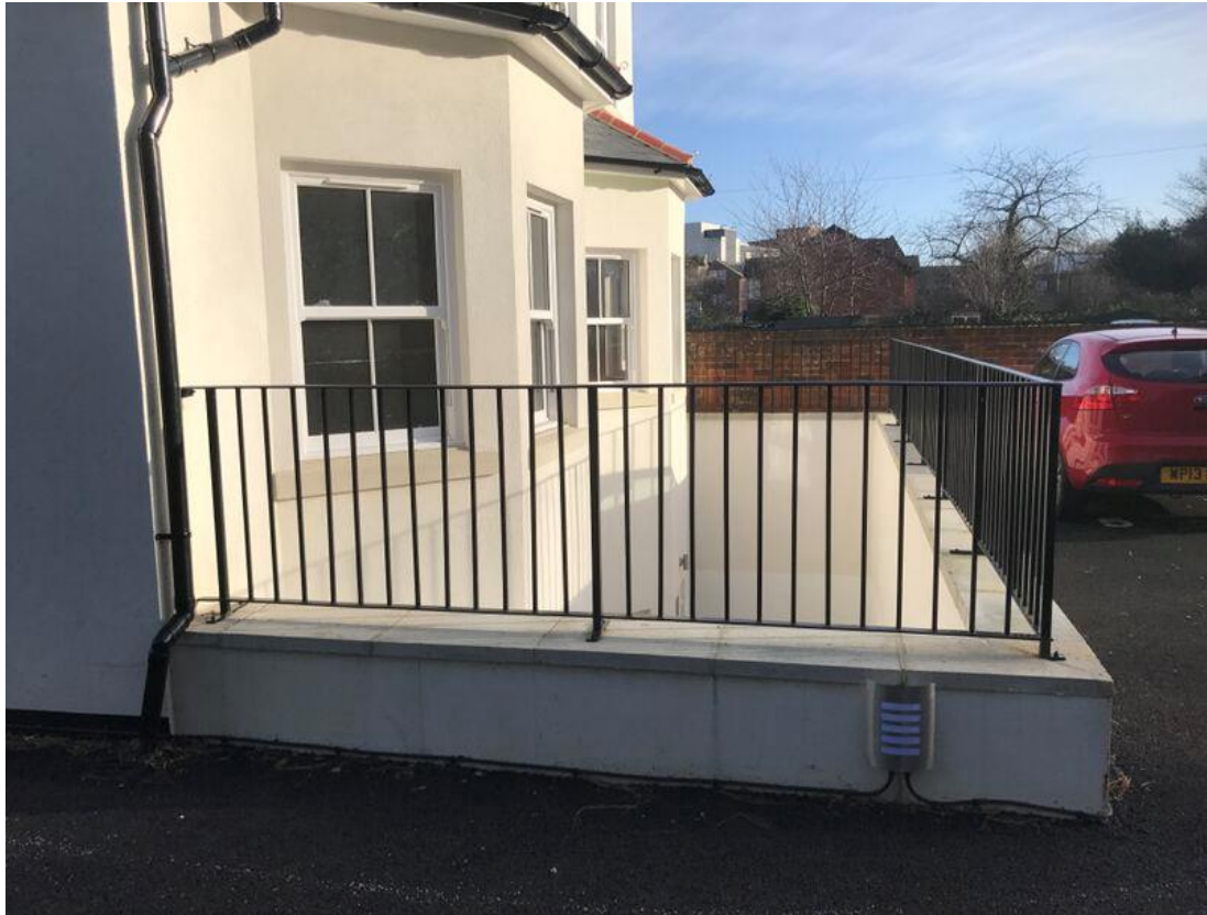
Existing rear lightwells to rear elevation
