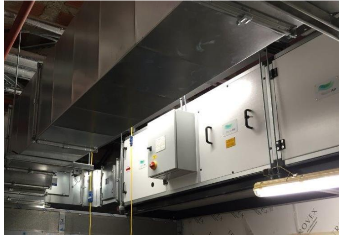
RA1.5 Ceiling Void
