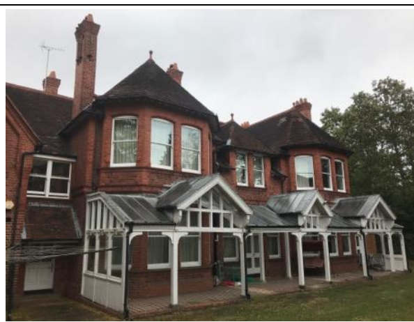
Photo 4 – Eastern end of southern elevation
