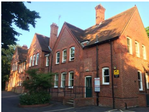
Photo 1 – Western end of northern elevation
