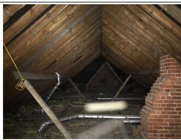
Photo 12: Inside felt lined section of loft
