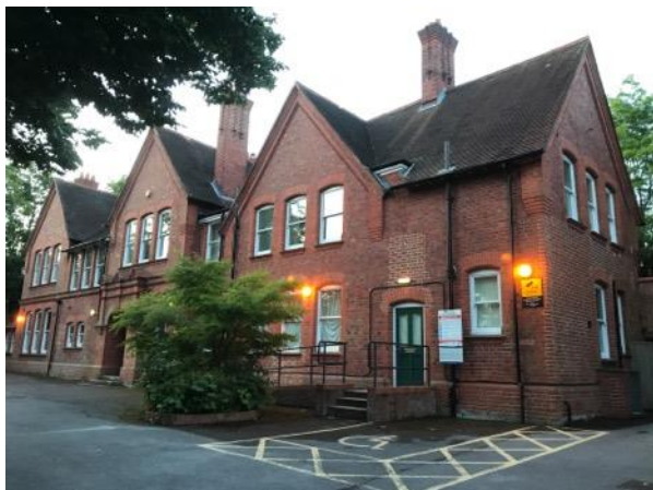
Photo 14 – Western end of northern elevation
