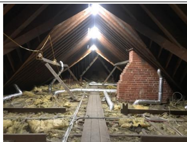
Photo 19: Interior of loft space
