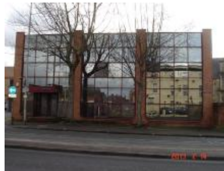
Existing building at 125 Chatham Street
