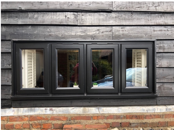
Photo 5 – Kitchen window replaced as part of the 2019 works, provided for comparison purposes
