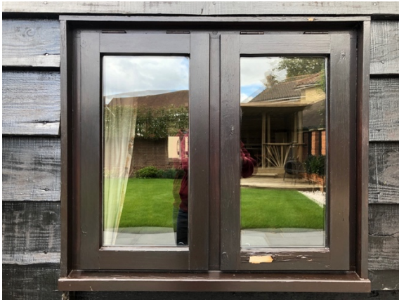
Photo 1 – Lounge window to be replaced
