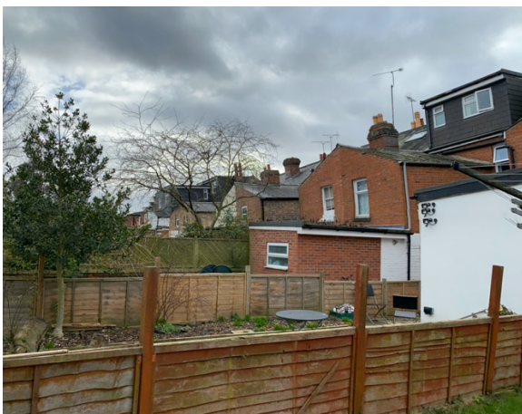
Juxtaposition of various extensions and lofts seen along the street
