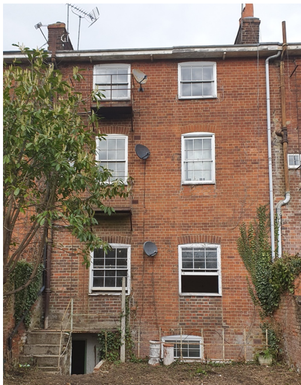
Figure 2:: 245 Oxford Rd-rear-Existing photograph
